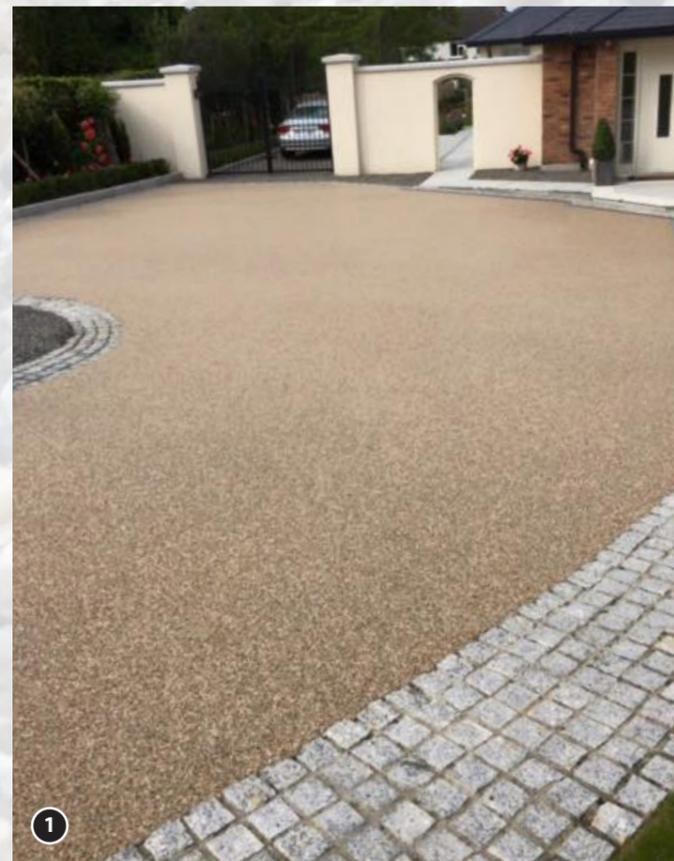
Factors effecting choice are: colour, hardness, texture. Pathways can use all but the softest aggregates: drives will require pea gravels, granites or basalts which are more durable. Steep drives will require an angular aggregate to ensure good grip, whilst a drive likely to have children playing around, may require a rounded pea gravel.
